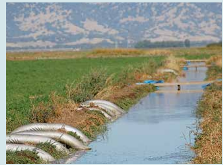
Siphons direct water from an irrigation ditch into the furrows of an alfalfa field.
